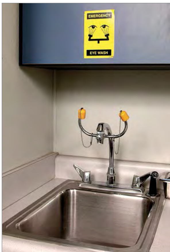
For worker safety, a euthanasia room should ideally contain an eye wash station
